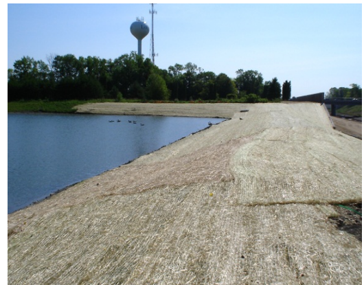
Erosion control blanket stabilizes pond slopes.
