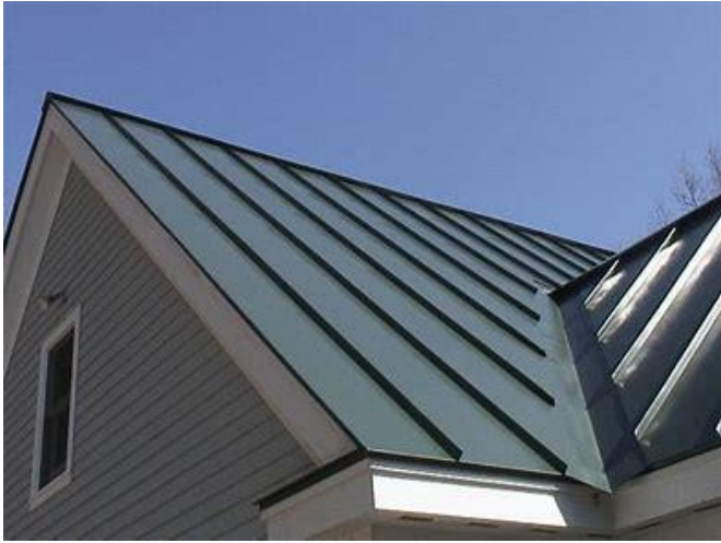
Example of a 1.5" Standing Seam Metal Roof
